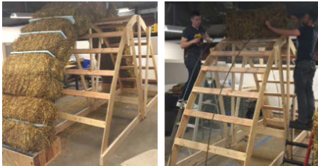
B8. Prototypes for hay bale loft construction intended for Mongolian school design. R. Whitehead studio, Spring 2015.
