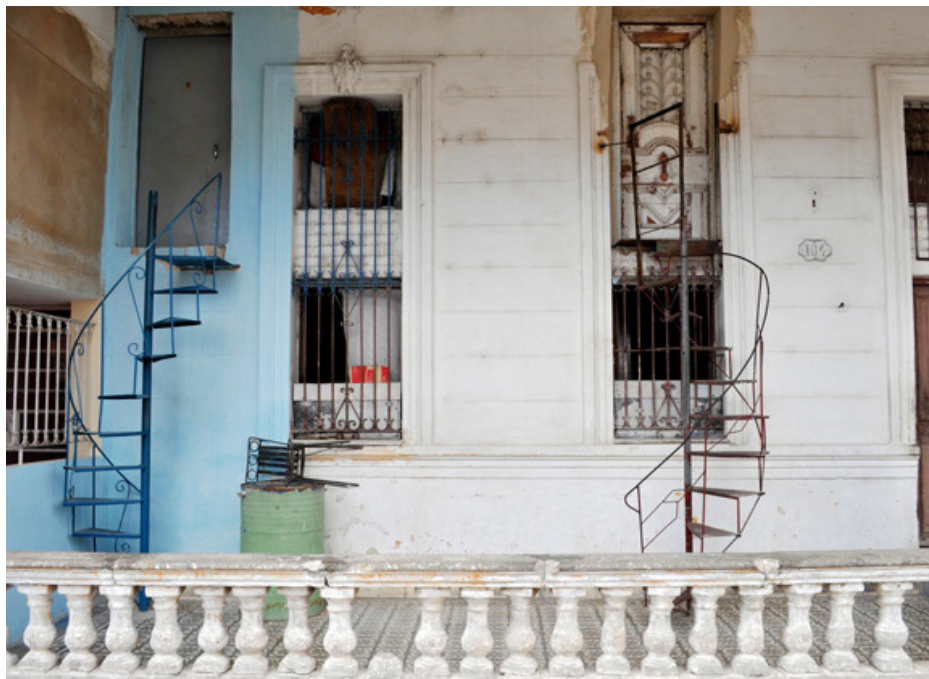
15. To circumvent building code, non-compliant stairs lead up to a storey addition that can remain alegal / Oroza 2006
