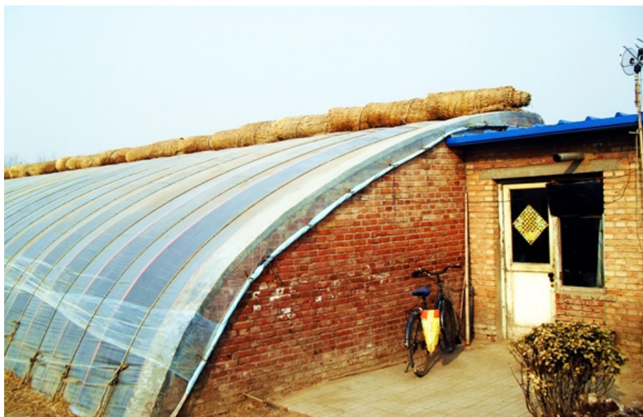
20. A solar greenhouse with thermal massing allows cold-climate farming in China / Buhler 2014
