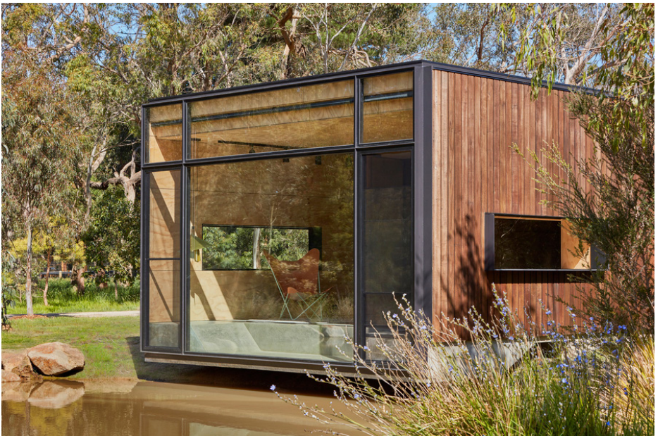
3. A modern low-tech house that uses water and convection currents for passive cooling but looks very different to vernacular architecture / Clarke 2017
