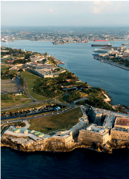
B3 Havana Bay Tunnel east portal
