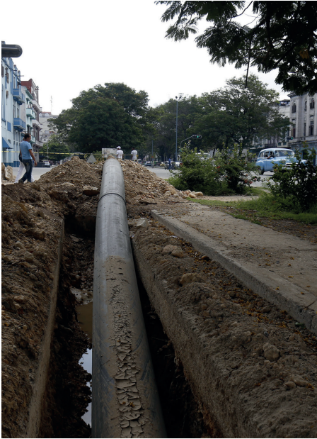
B1 Water supply replacement with MDPE pipe
