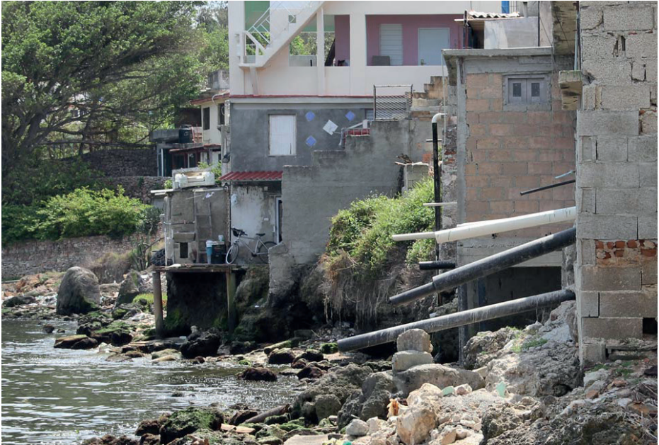
B7 Sewage outflows discharge directly to the sea in some cases
