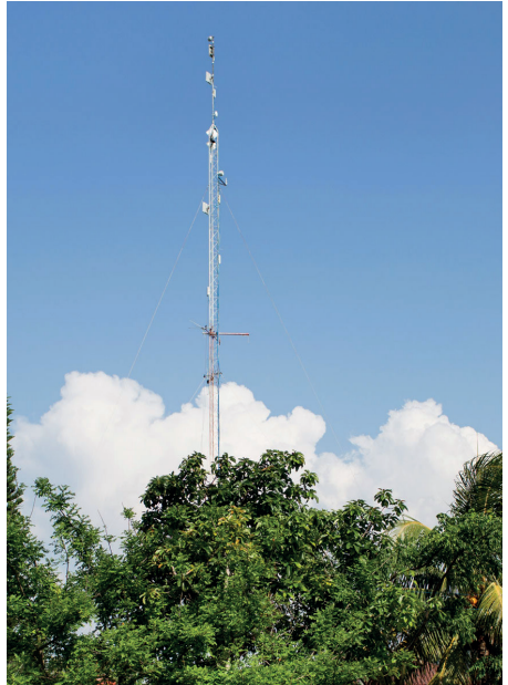
B2 SNET pilar (antenna) as part of domestic intranet
