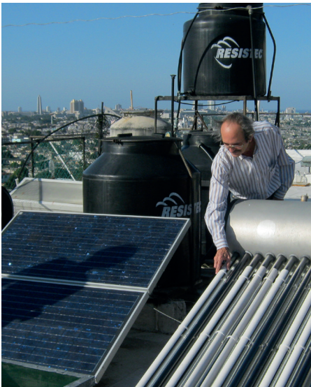
B19 Luis Bériz's power plant on a roof of Havana
