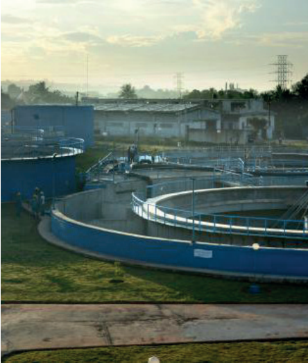
B9 Settling tanks at a new wastewater treatment plant
