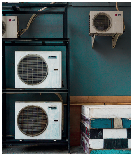
Typical setup of cooling systems / Source: Unsplash
